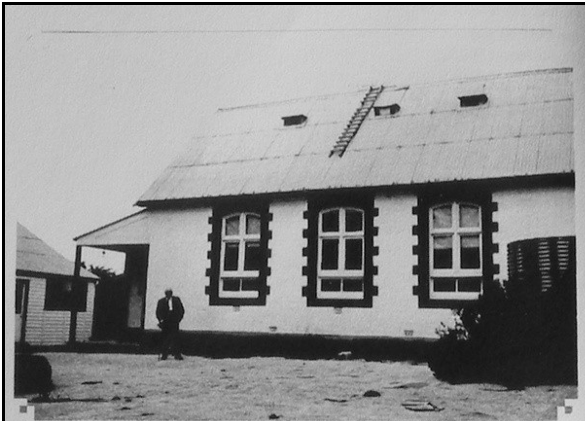
The school we attended at Beachport, James Chant in the foreground. The building is no longer used as a school (1983)
